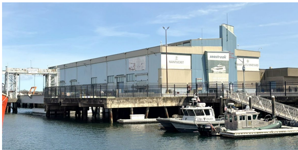
Public safety marina, Seastreak berth, and existing warehouse at the State Pier.
