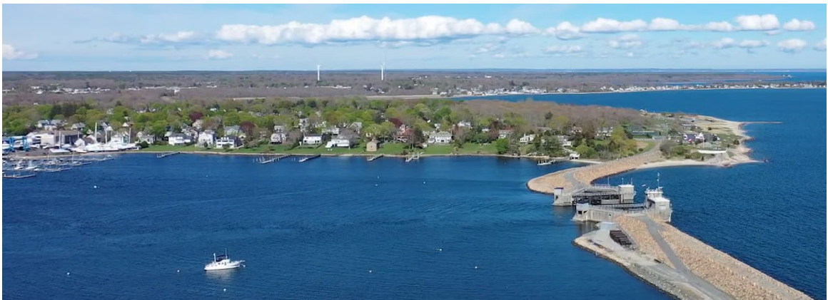
Fairhaven Waterfront and New Bedford Hurricane Barrier.
