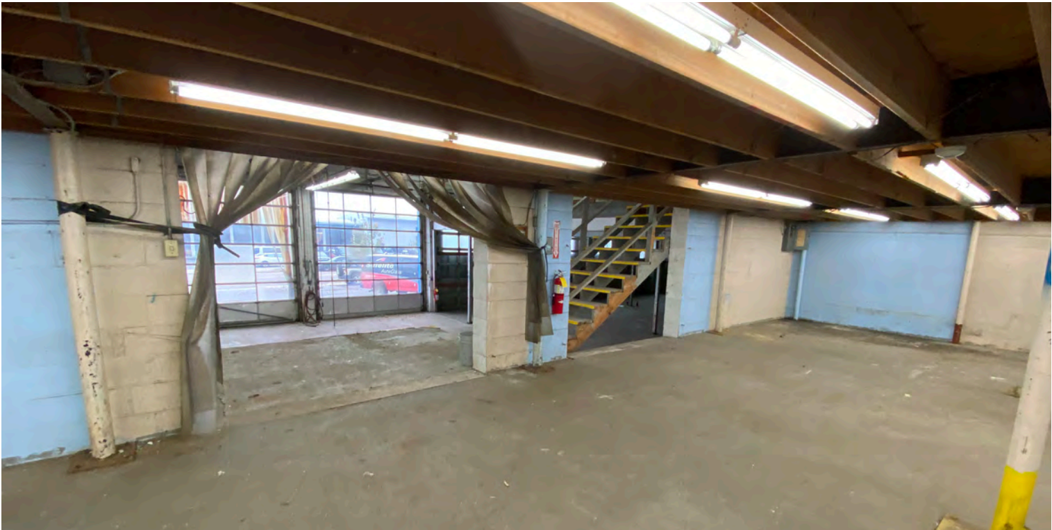
VIEW FROM PARTIAL FLOOR UNDERNEATH EXISTING STORAGE MEZZANINE. CEILING HEIGHT TO UNDERSIDE OF STRUCTURE IS +/- 6' - 7" (STORAGE ABOVE IS +/- 4' - 11" TO UNDERSIDE OF STRUCTURE).
