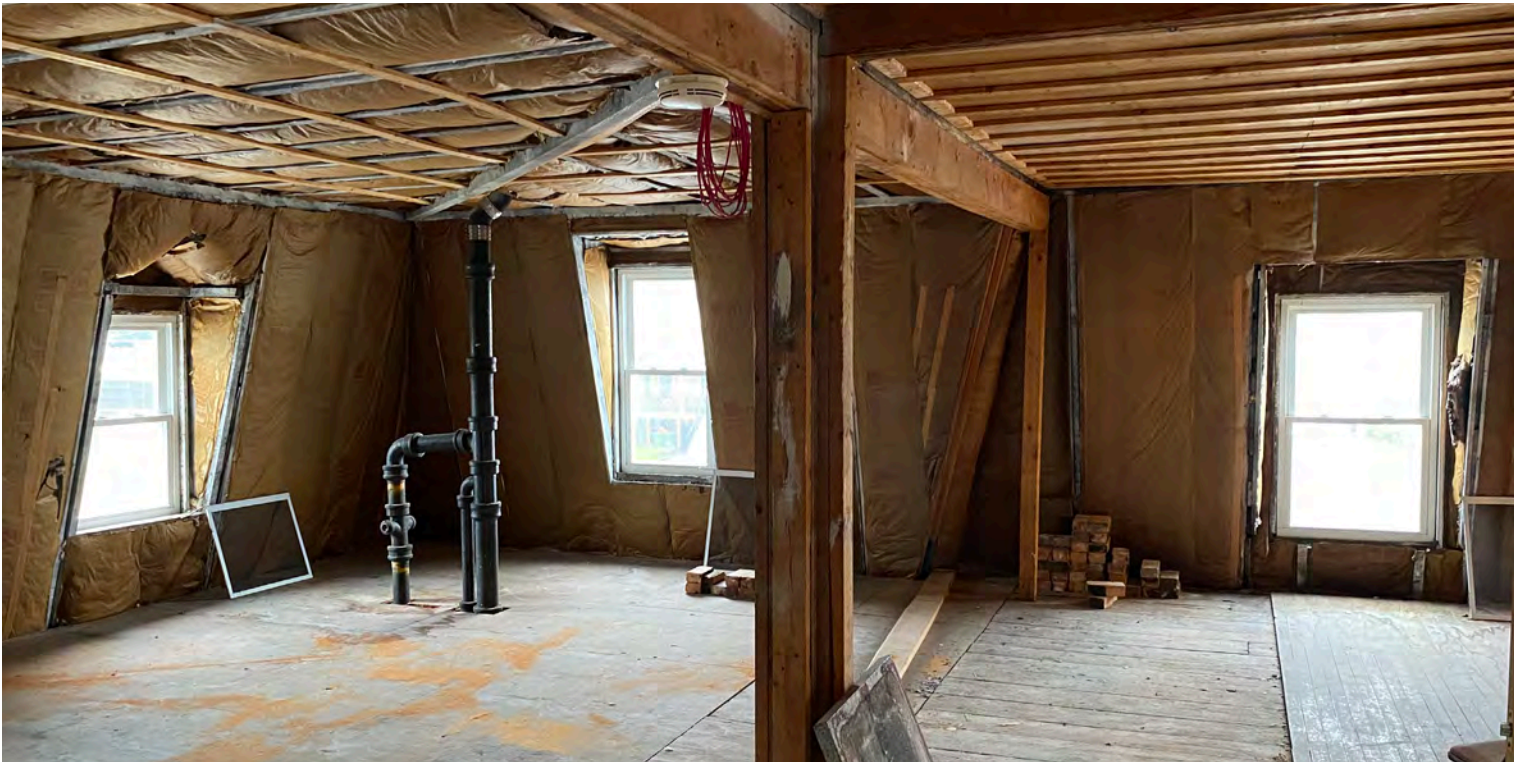
THIRD FLOOR OF 'BUILDING 4' WHERE SOME PARTIAL RENOVATION WAS DONE, INCLUDING WINDOW REPLACEMENT, INSULATION INSTALLATION, ETC.
